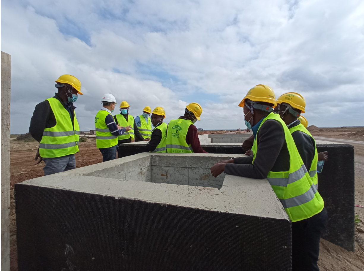
Top view of the tunnels
