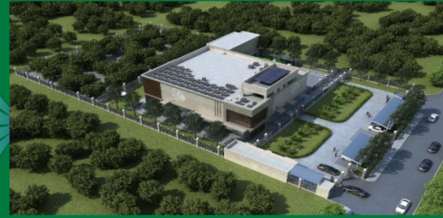
Phase2 Primary Data Center Construction time: November, 2019 - October, 2020
