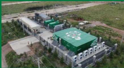
Phase1 Data Center / DR Construction time: March, 2019 – May, 2020
